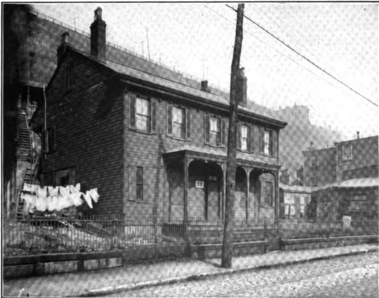
TENEMENT OF OLD DWELLING TYPE It is these old one-family houses, converted into shelter for 3 or more tenant families, that present the most exacting problem of regulation and inspection
