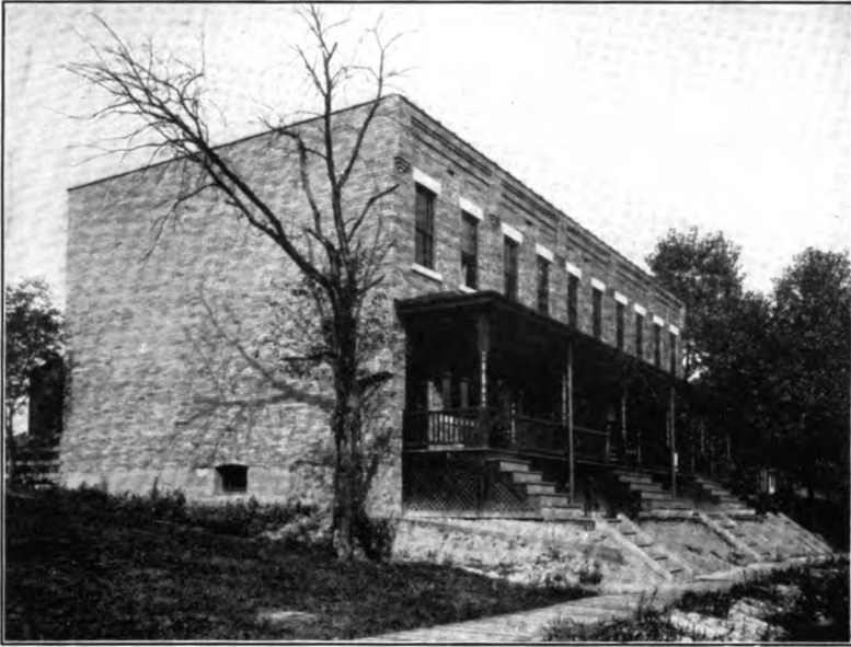
ROW OF FIVE NEW ONE-FAMILY BRICK HOUSES Five rooms in each house; bath tub and closet; sink in kitchen. McKees Rocks
